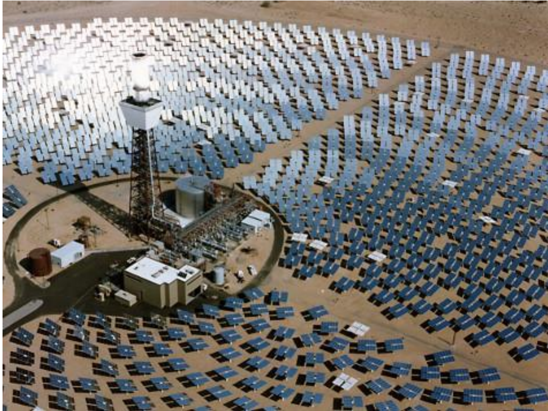
Figure 8 Solar thermal plant [48]
